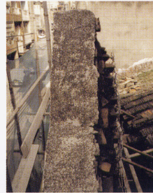
如意形山牆牌樓面背後之火頭磚。 Poorly baked bricks behind the gable of the façade of the arcade
