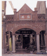
協興的清水磚牌樓立面。 Façade of the arcade of Sie-sing made of red bricks
