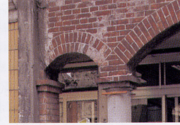
牌樓面間柱的磚圓拱及磚疊澀柱頭。 The pillar capital built of layers of bricks with each layer projecting from the previous layer and the brick circular arch
