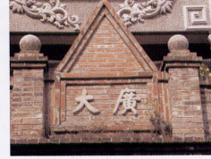
灰泥凸縫的磚縫作法是土水師傅拿手的功夫。 Protruding seams made of plaster between layers of red bricks, a mastery skill of the builders
