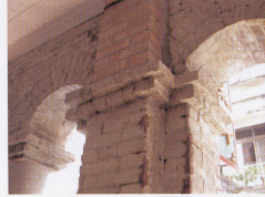
亭仔腳共同邊柱的磚疊盪柱頭。 The pillar capital built of layers of bricks with each layer projecting from the previous layer in the arcade
